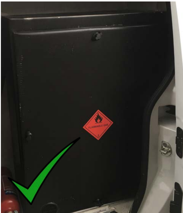
Example of a transport storage locker.
